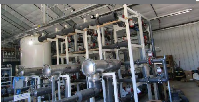
CRESTED BUTTE WTP IMPROVEMENTS
