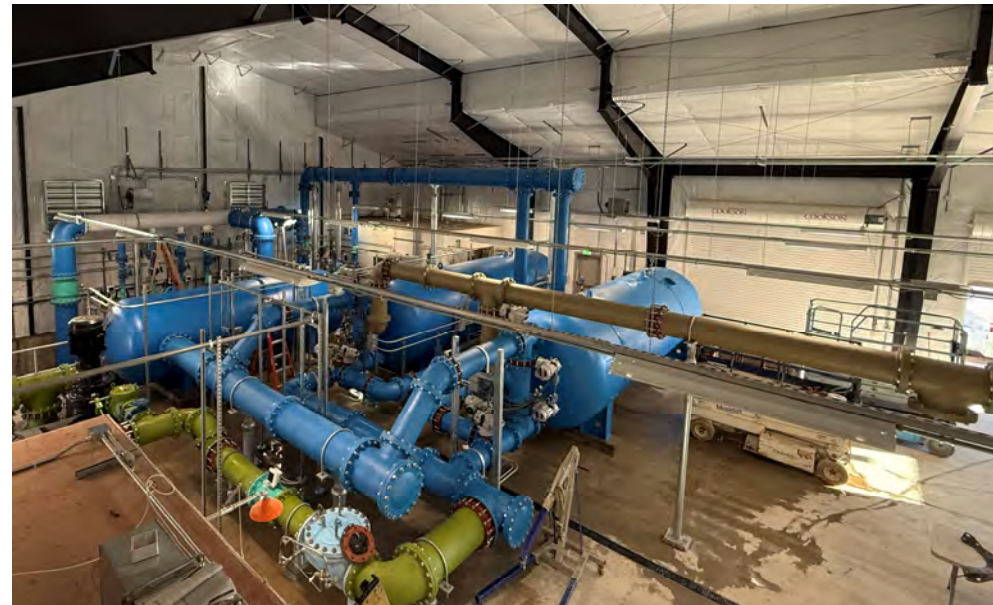
Sterling Ranch Water Treatment Plant
