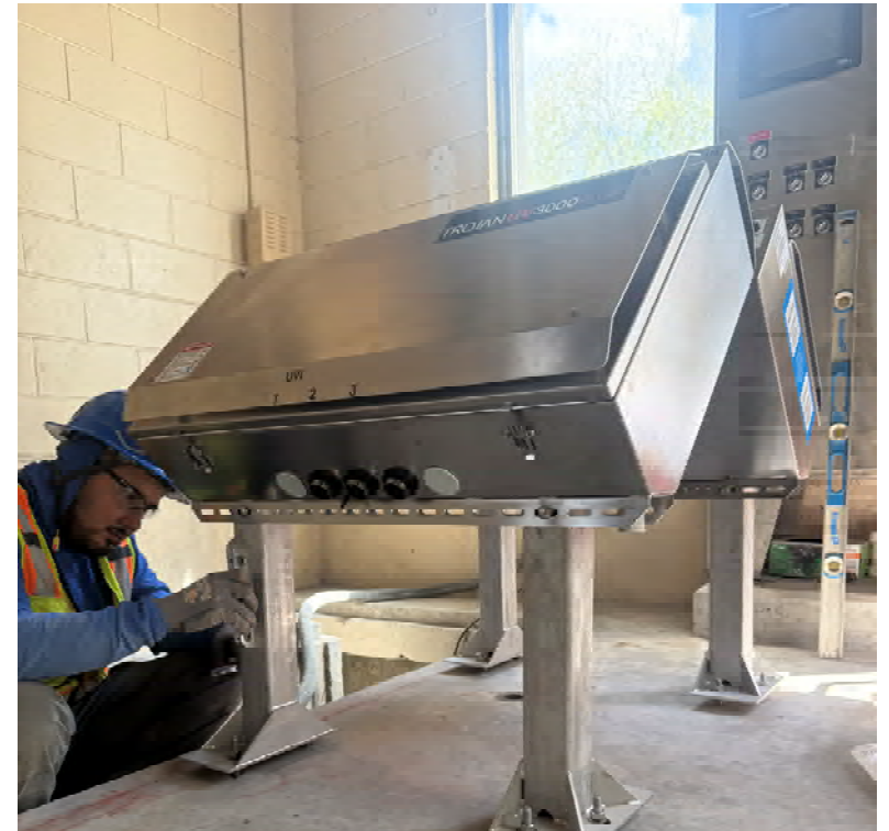
Montrose Wastewater Treatment Plant
